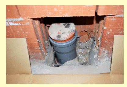
Examples of inapplicable sealing around pipe penetrations
