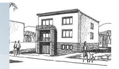
Houses were built in period of 1972-1983 and distributed over the whole country (mostly around Prague), high levels of indoor natural radioactivity identified in 1987 in walls construction material (slag concrete panels with high concentration of **Ra-226**)
