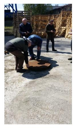
Closed down in 1966: backfilled with use of flyashe and covered by reinforced concrete cover. Measurements are performed in the office of company located near the shaft.
