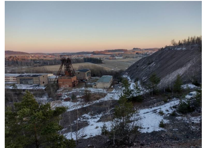
View of Shaft 15 from top of the dump, Original photo
